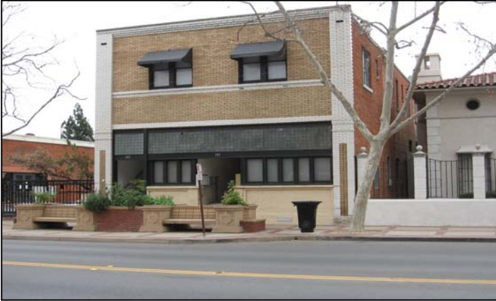
78 Dwelling Units/Acre (183-185 S. Glassell) 7 units on a .09 acre site
