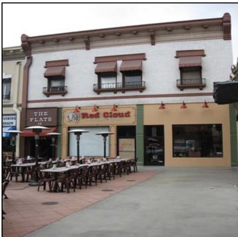
29 Dwelling Units/Acre (38 Plaza Square) 10 units on a .34 acre site
