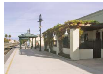
Orange Metrolink Station
